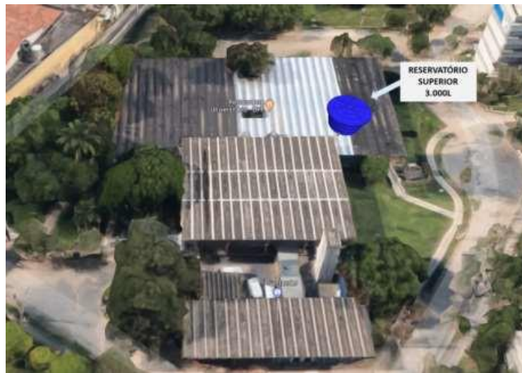
Figure 2. Schematic drawing to exemplify the position of the upper reservoir. Rio de Janeiro, 2018. Source: Adapted from Google Earth.
