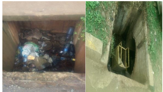
Fig. 2. Photos of the waste deposition in drainage infrastructure.
